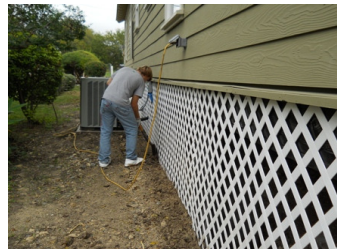
Will trenching around the HOTC7
