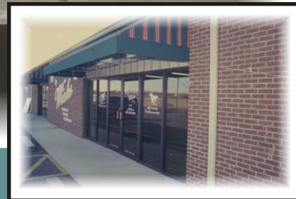
Firebaugh Complex; Sargent Construction Co. builder.
