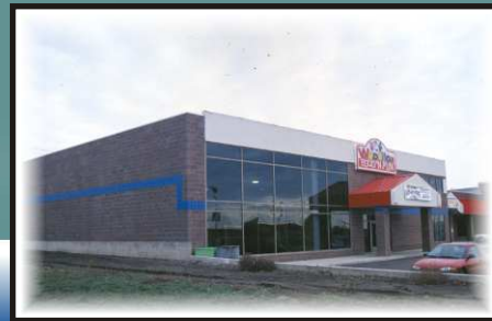
Above, Metro Center; Northstar Steel, Inc., builder; Hoeffel Torno Nester Davison, architect.
