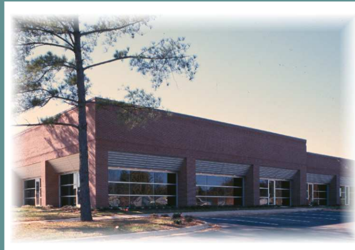
540 Commerce Center; Flythe Construction Company, builder; Truman L. Newberry, Jr., architect.
