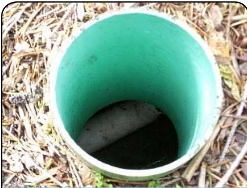
Inspection port dry on April 10, 2007
